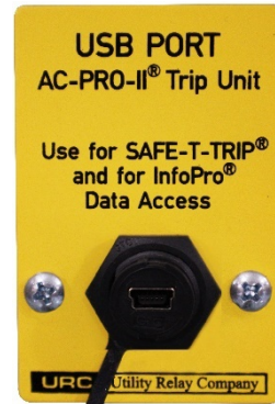
Cubicle door Mini-USB port (cover off) and legend plate
